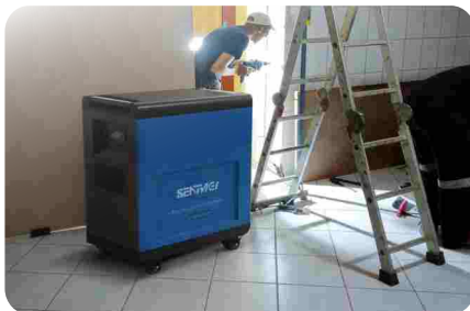
Drilling and Renovation
